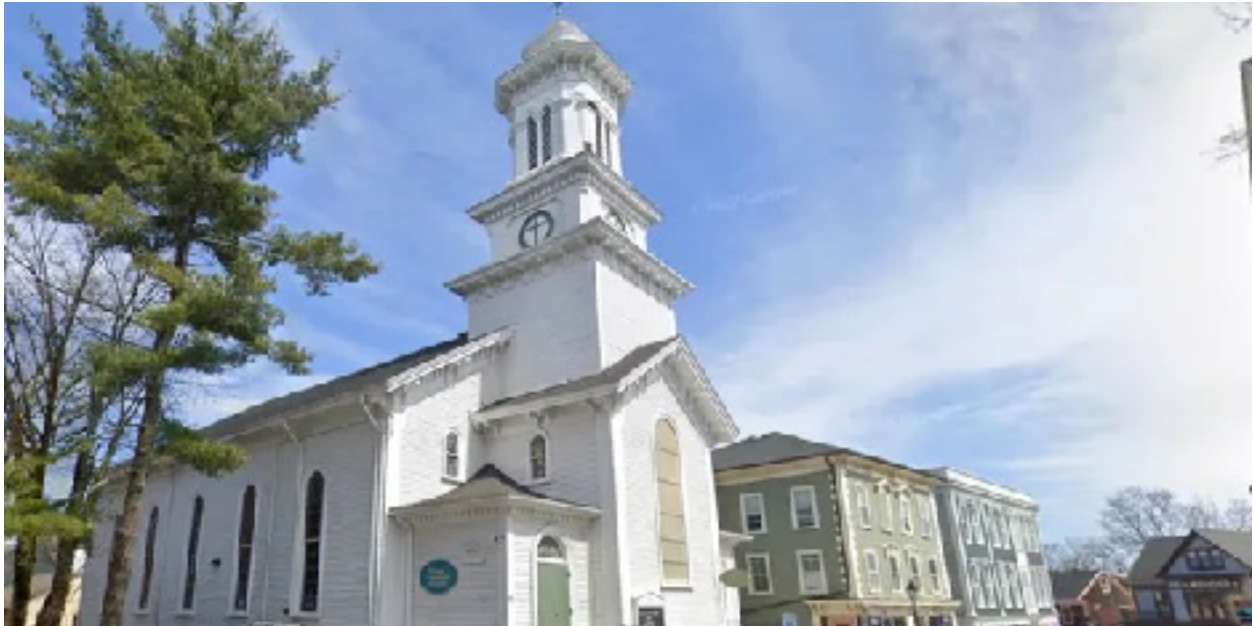
Grace Community Church in Marblehead, Massachusetts, was vandalized with graffiti. (Google Maps)
